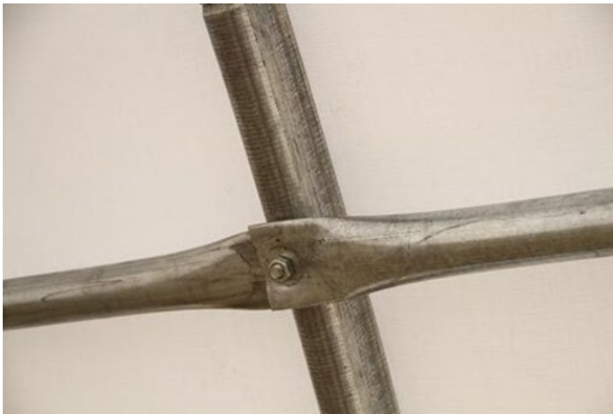
2) Connecting the Purlin to the Arch Tube
