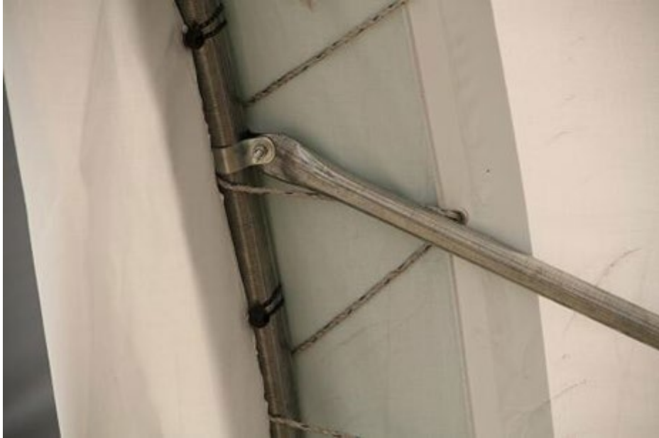
3) Installing the Diagonal Bracing Tube
